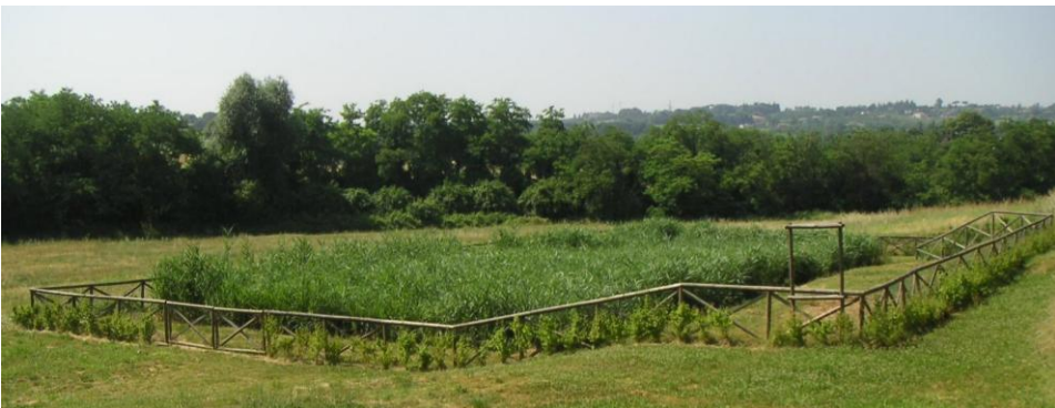
Figure 1-3: An example of a subsurface flow constructed wetland to treat urban wastewater for 362 p.e. in Ondrejov, Czech Republic.
