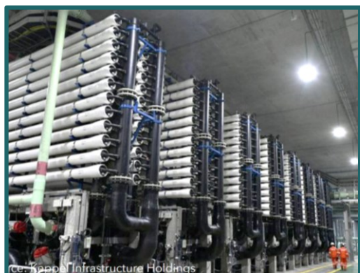
Figure 2. Reverse osmosis desalination plant (photography at the left), drawing water from the Marina Reservoir and the Singapore Strait. (IDA Desalination & Reuse Handbook 2021–2022, 2022). The reverse osmosis process (figure at the top) compared to the concept of osmosis occurring in nature.
