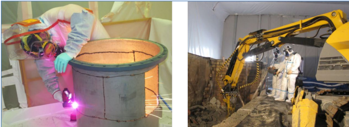
Figure 3.3.7-6. – Dismantling in confined space with PPE (left) and with a remote controlled excavator (right)
