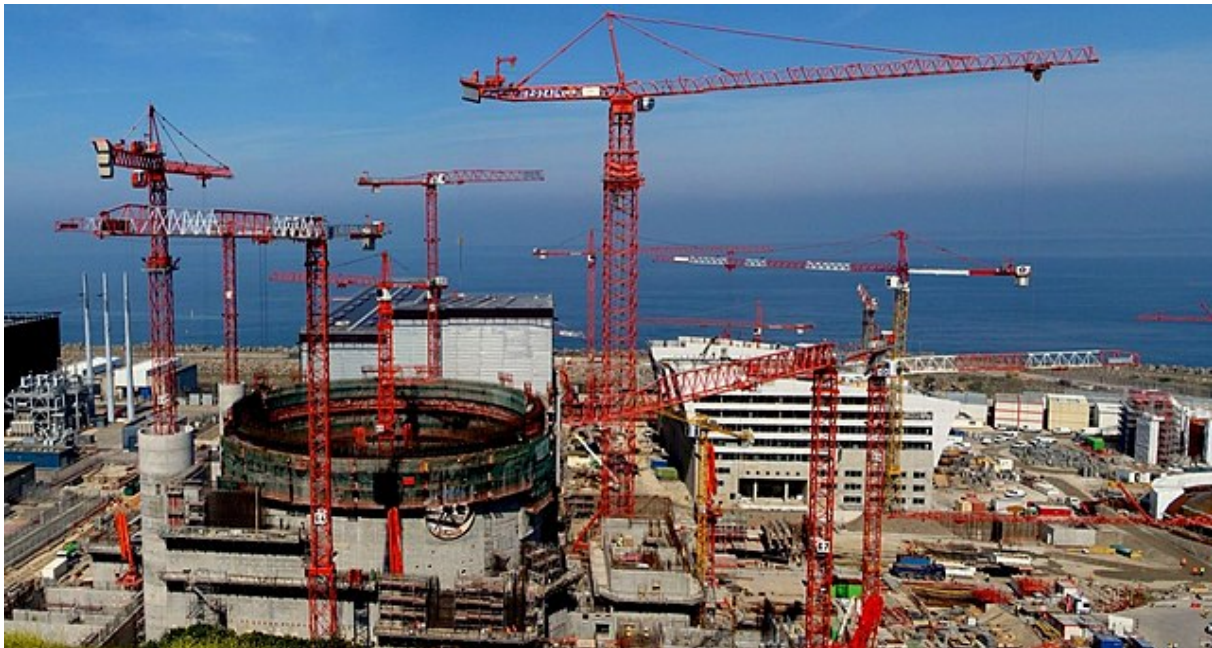
Figure 3.3.7-1. Unit 3 of Flamanville NPP under construction (France, 2010)
