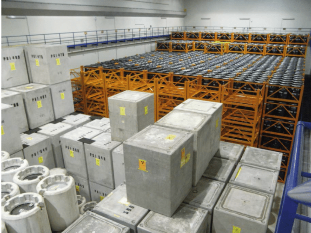
Figure 4.1-4. Interim low and intermediate level waste storage (Federal Interim Storage Facility, Switzerland)
