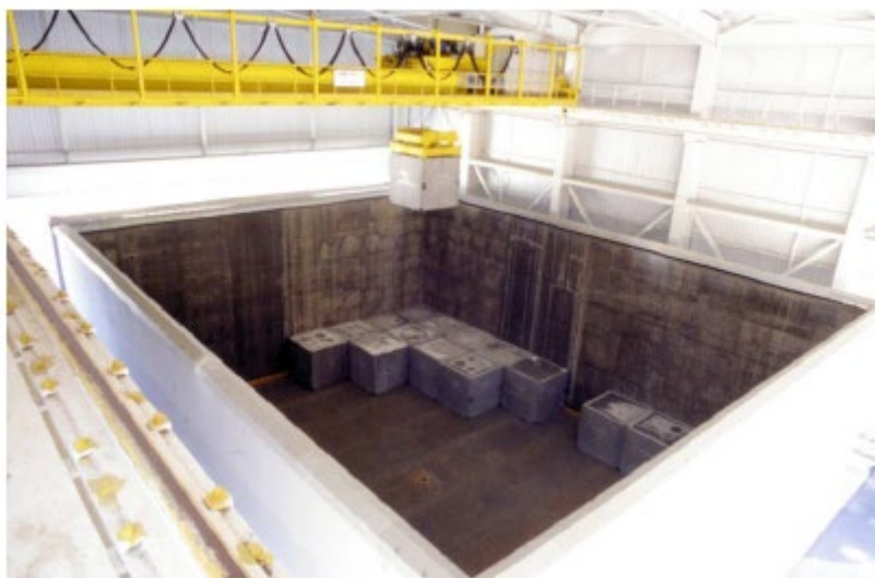
Figure 5.1-5. El Cabril near surface disposal facility, Spain.
