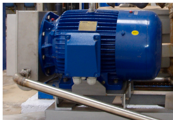
Fig. 2. Pelton turbine coupled with the generator.
